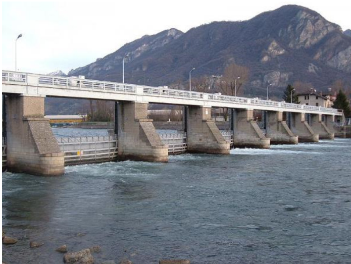
Figure 3.27: Figure 3.2.8: Olginate dam view from right site of the river.
