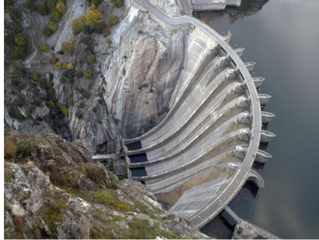
Figure 1.2.1. Aldeadávila arch dam (Spain-Portugal).
