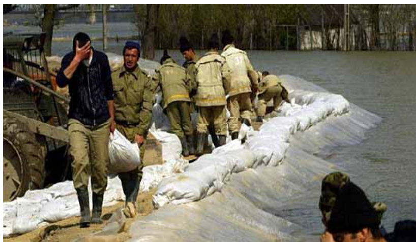
Figure 1.3.1. Settlement of sand sacks to reinforce dikes in Rumania in 2006.
